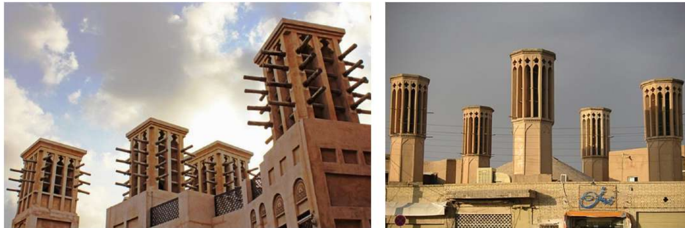
figure 4 . A traditional windcatcher is based on a simple technique. Porous pots of water convert dry air into humid air, and charcoal on a grating increases the flow of air into indoor spaces. Here, indcatchers were only used to affect the inside of buildings
