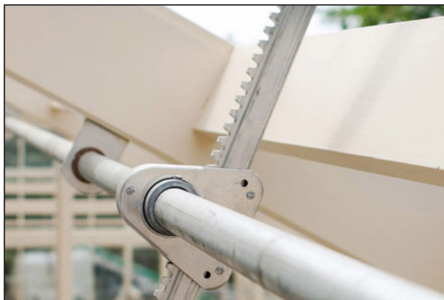
Rack & Pinion Vent Actuators (Climate Controls, 2023)
