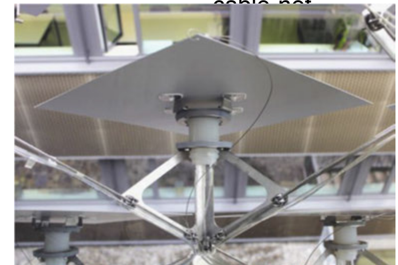
Cantilever design with double bent and laser-cut stainless steel (Nagy et al., 2016)
